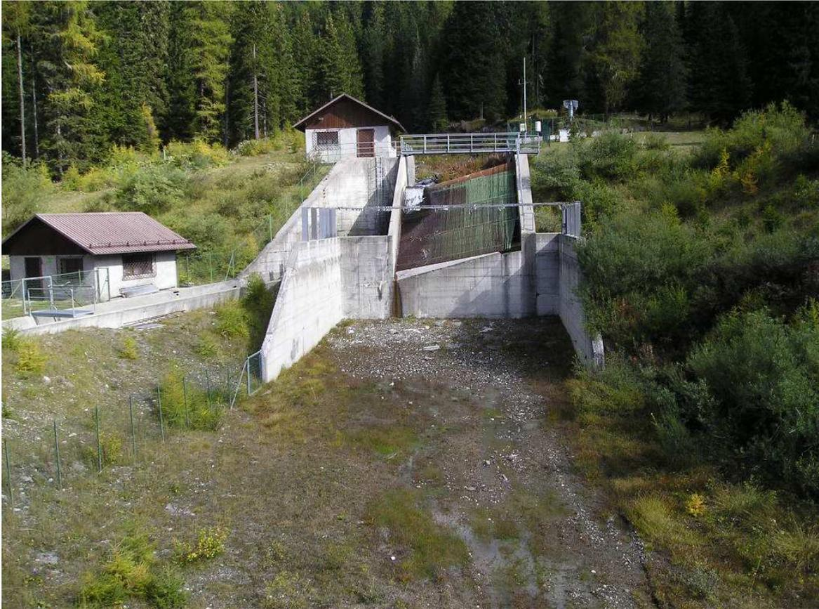
**Figure 4: ARPAV's solid discharge measuring station (upstream part)**
