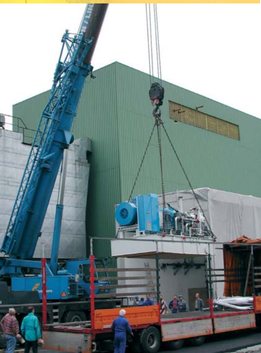
Installation of SSE
