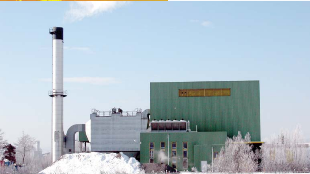
Biomass CHP plant Hartberg - water tube steam boiler (18 MW th ), CHP module (710 kW el ), dry electrostatic precipitators
