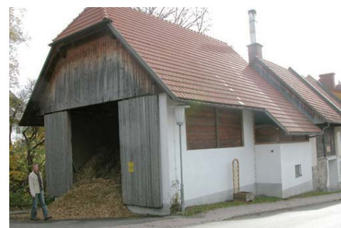
St. Oswald: store with boiler house
