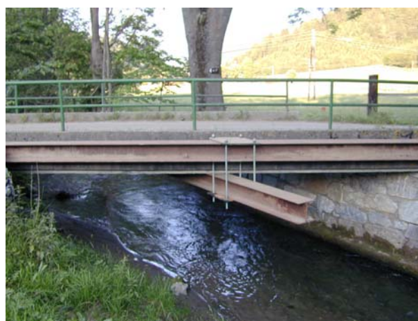
Fig. 14: Reinforcement of a bridge in Oberzeiring
