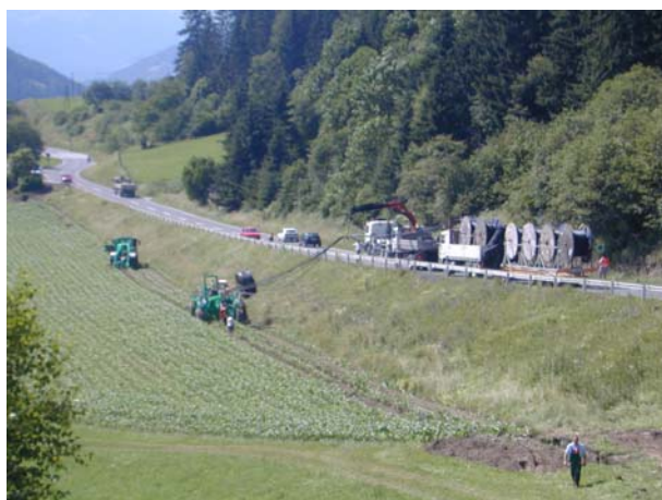
Fig. 24: Installation of cables in Oberzeiring using ploughs
