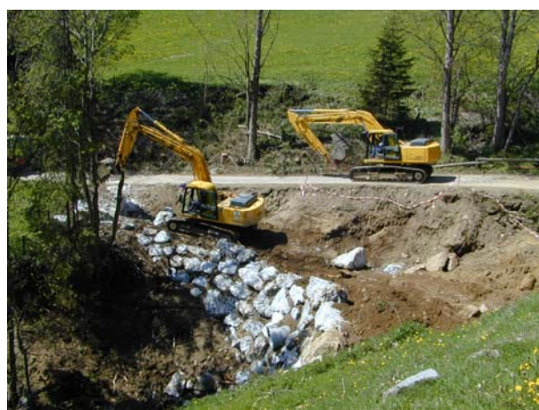
Fig.13: Widening a bend in Oberzeiring (A)
