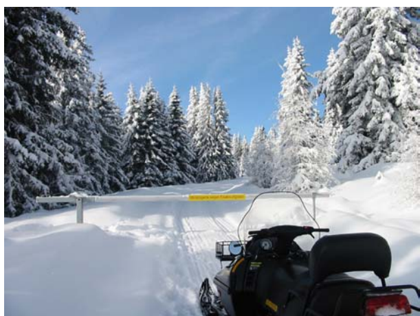
Fig. 47: Road barrier when there is danger of falling ice
