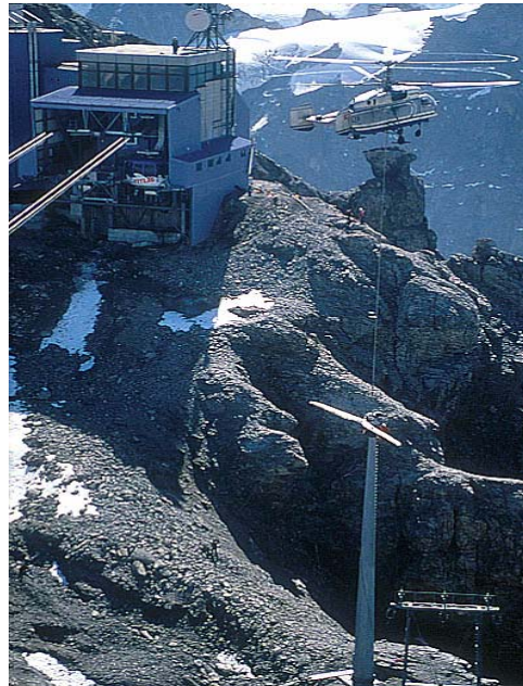
Fig. 19: Transport of a wind energy plant with nacelle and rotor to the Chli Titlis (CH) site at an altitude of 3,000 m
