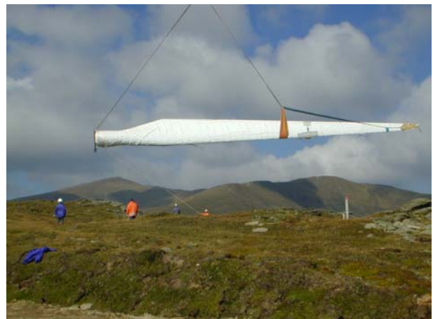
Fig. 22 Transport of rotor blades by helicopter in Oberzeiring (A)
