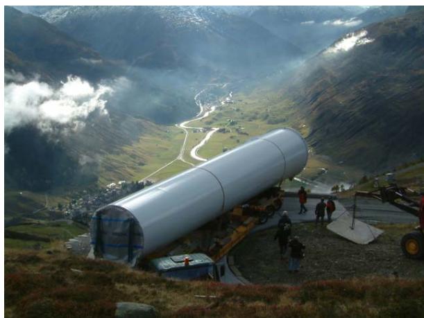
Fig.17: Transport of a tower segment up to the Gütsch (CH)
