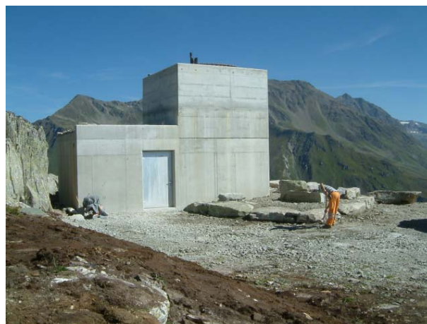
Fig. 28: Foundations with incorporated transformer station on the Gütsch (CH)
