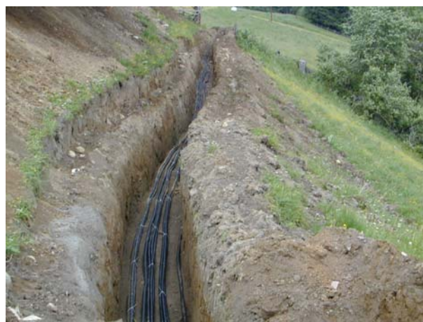
Fig. 25: Installation of underground cables in awkward and steep terrain in Oberzeiring
